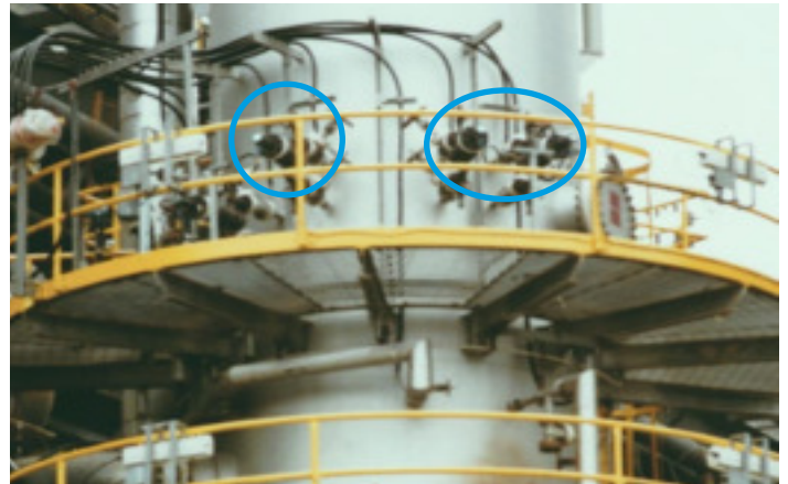
2 high and 1 high high alarm
