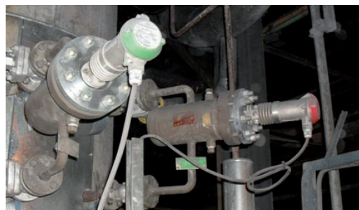
Trimod Besta level switch type: HAA 22C01 041 Trimod Besta float chamber type: I021-1C0RC1
