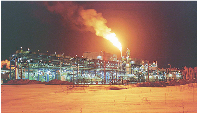
Fuente: Luginetsky Gas Compressor Station Strezhevoy, Siberia occidental, Rusia
